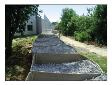
Photograph 4.5 Gravel Filled Containers that Form a Flood Barrier
