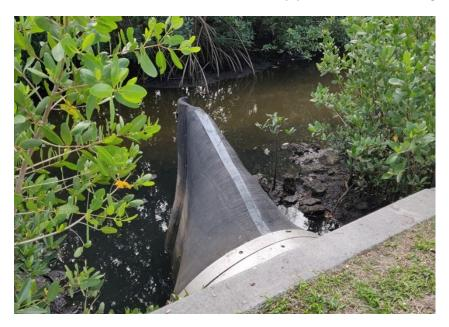
Photograph 4.3 Stormwater Check Valve for Backflow Prevention
