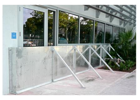
Photograph 4.7 Temporary Flood Barrier Protecting Building Entryway (http://www.flood-barriers.com/floodpanel.html)
