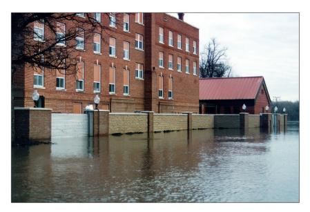
Photograph 4.6 Masonry Floodwall with Engineered Temporary Flood Gates (FEMA, 2013)
