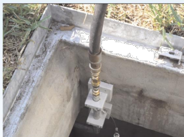
HydroSlide® quick connector with vacuum truck water supply hose attached for debris removal.
