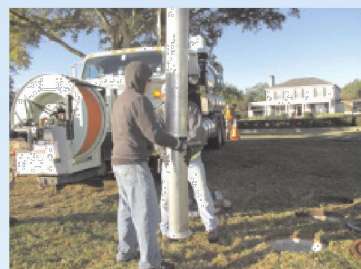
The use of a vacuum truck allows for easy debris removal without entering the structure.
