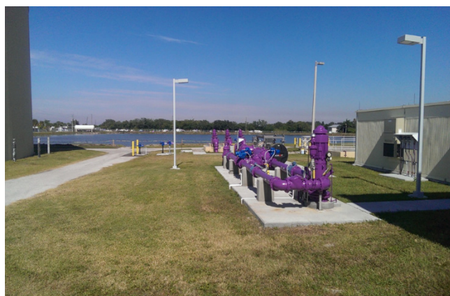
Completed Reclaimed Water ASR Wellhead facility with ultraviolet disinfection treatment and sodium bisulfite pretreatment.
