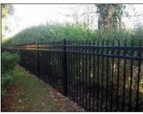
RAILING IS TO BE 42" HIGH ALUMINUM PICKET, COLOR IS TO BE BLACK POWDER COATED FINISH WITH PRESS POINTS ON %" SQUARE PICKETS WITH CIRCLE CAPTURE DOUBLE TOP RAIL, 2" SQUARE POSTS AT 6" SPACHIG, CONTRACTOR TO PROVIDE ENGINEERED SHOP DRAWNICS.
