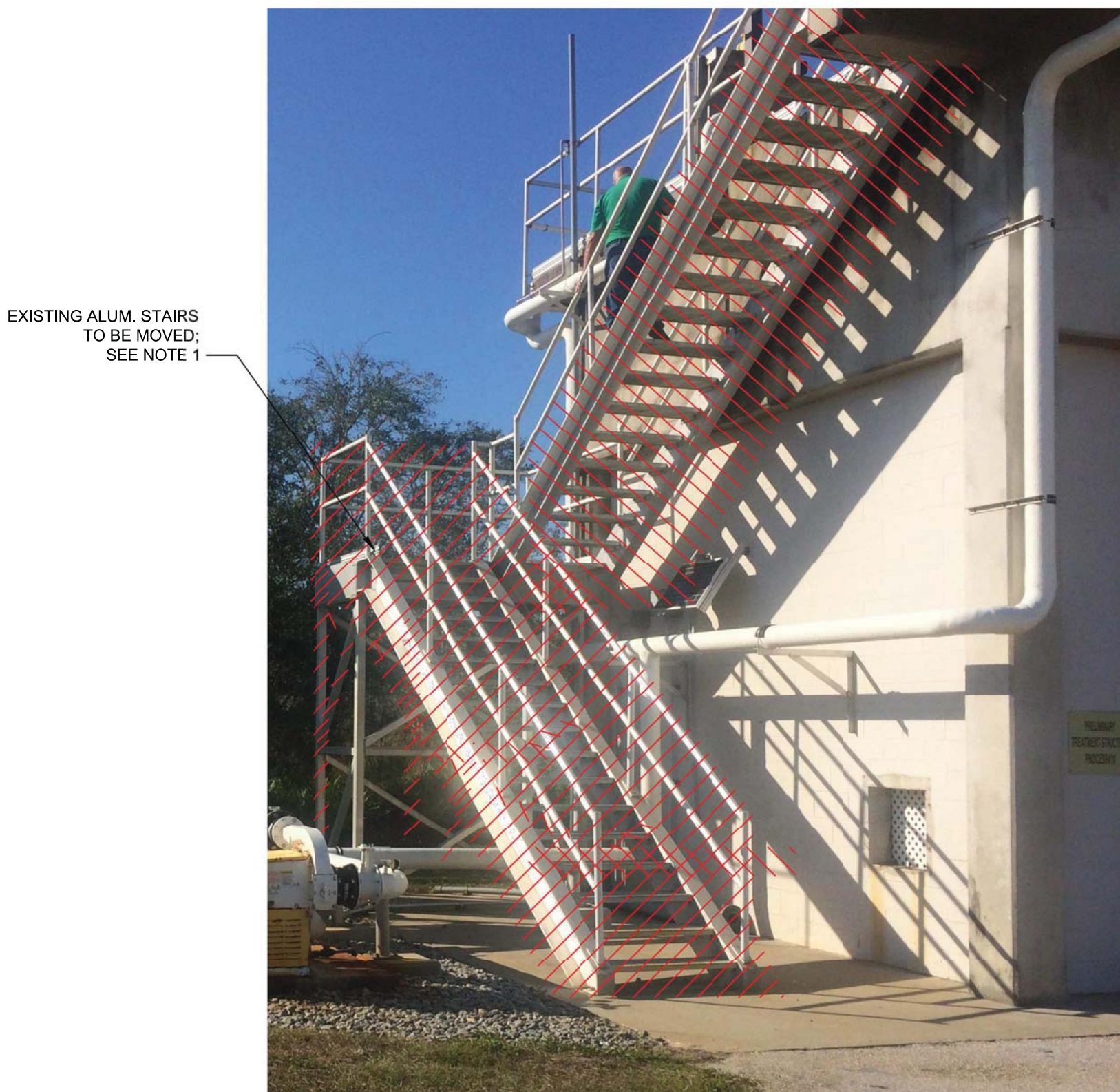
NOTE: 1. EXISTING ALUMINUM STAIRS ARE TO BE DISASSEMBLED AND REASSEMBLED AT THE NEW LOCATION; SEE KEY PLAN.
