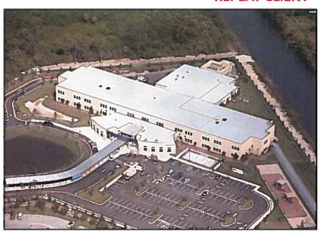
GATES constructed Mike Davis Elementary School for The District School Board of Collier County on schedule and on budget. The 117,000 SF, 2-story building was constructed using the tilt-wall construction system, structural steel frame, metal and built up roofing, with all interior drywall finishes. Other scope requirements included classrooms, kitchen, cafeteria, administrative offices, the bus loop, site work, playground areas, parking lots, and walkways.
