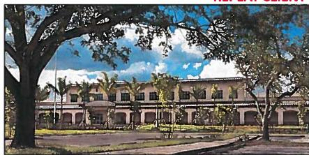
The new 195,048 SF facility was constructed on 23.41 acres. Construction consisted of exterior concrete tilt-wall construction with structural steel frame and low-slope roofs. The facility is capable of withstanding a Category 5 storm event with emergency generator power to accommodate critical building systems for continuous operations.
