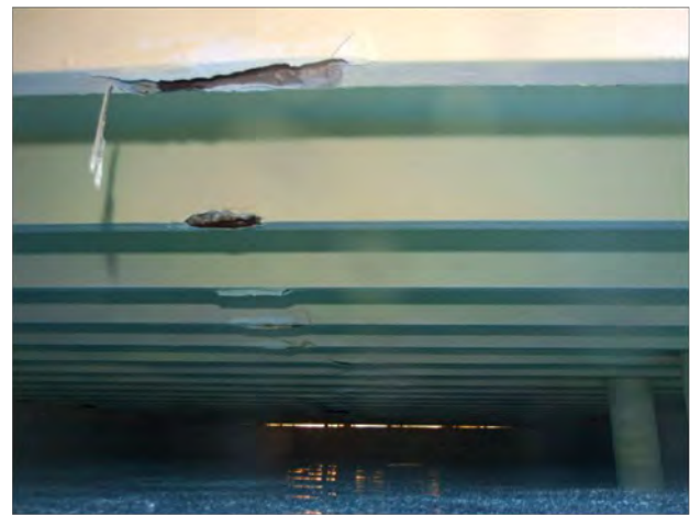
TYPICAL SPALL PHOTOS
