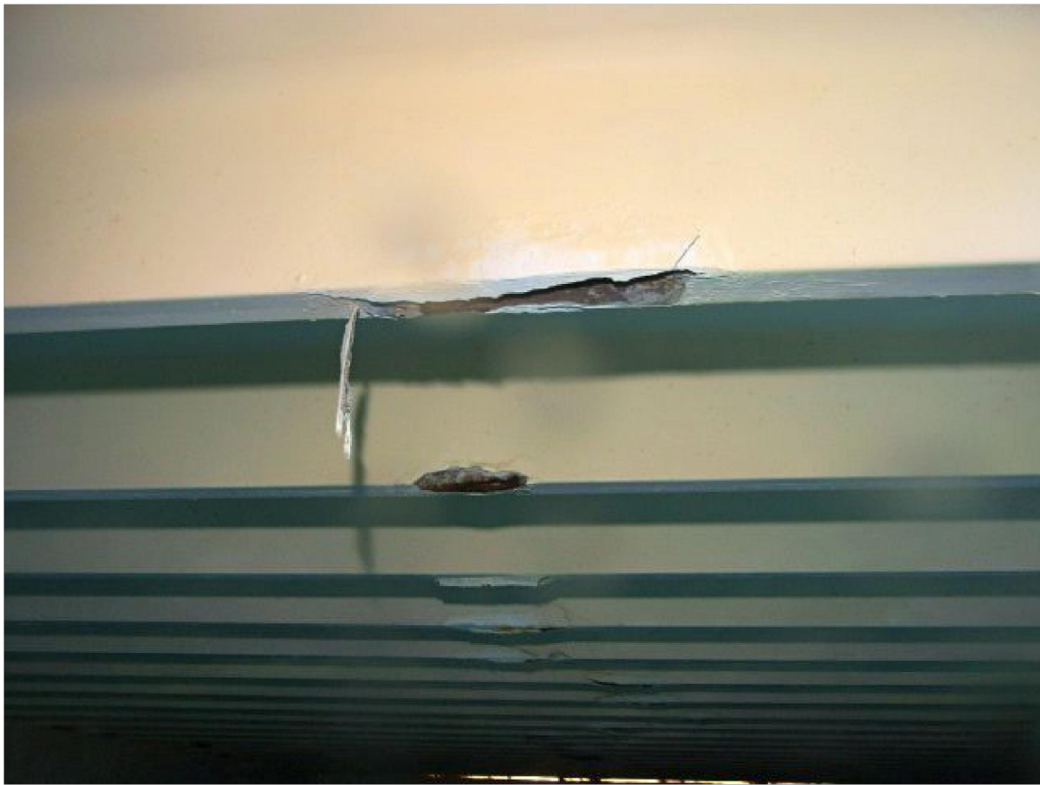
TYPICAL SPALL/EXPOSED REINFORCING PHOTOS
