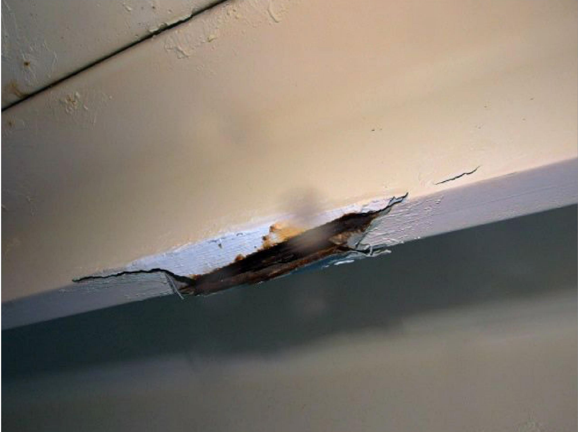
TYPICAL SPALL/EXPOSED REINFORCING PHOTOS
