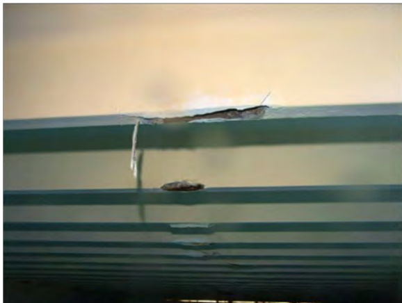
TYPICAL SPALL/EXPOSED REINFORCING PHOTOS
