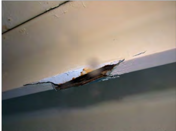
TYPICAL SPALL/EXPOSED REINFORCING PHOTOS
