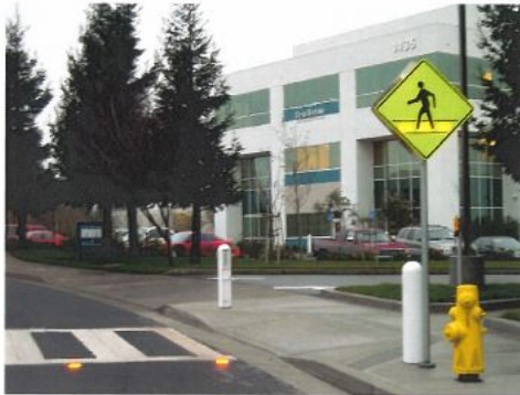
Smart Crosswalk with motion activated flashing lights (LightGuard)
