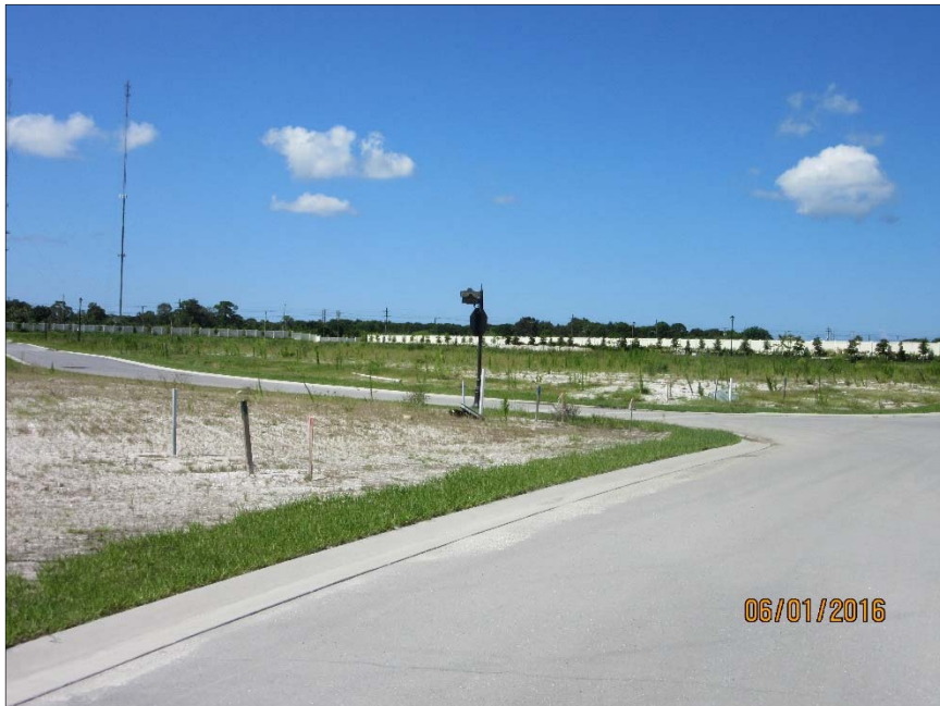
View of Unit 1, Phase 4 looking south toward Laurel Road. Pescador Place is the street in the foreground.
