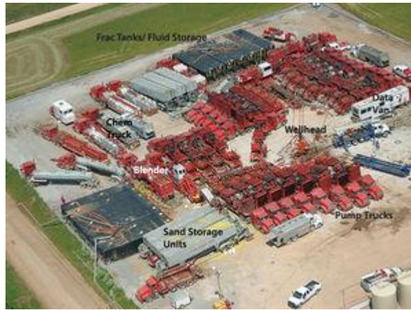
Aerial view of an hydraulic fracturing site
