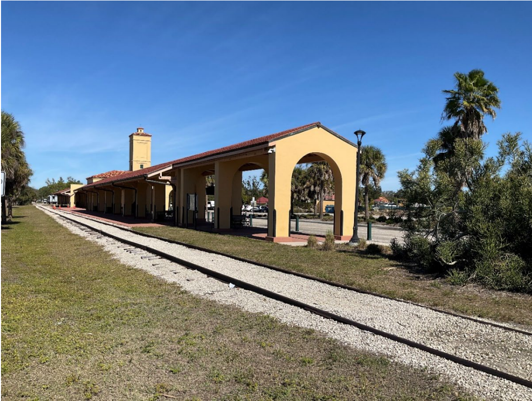
Figure 5-7. Venice Depot, 303 East Venice Avenue (S000585), facing east.
