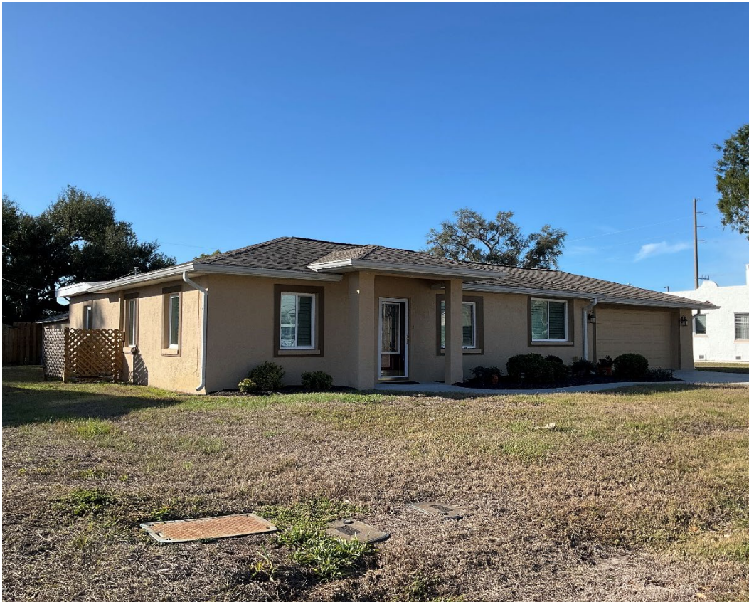
Figure 4-11. A Ranch style resource at 720 Myrtle Avenue (S019080) in Edgewood.
