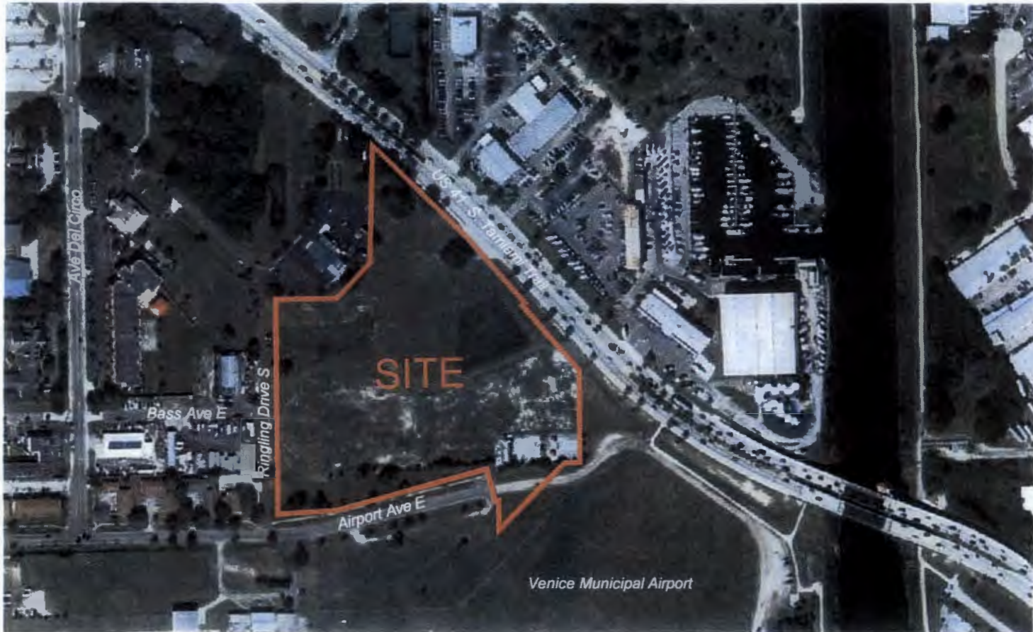
The 11.5-acre Ringling Park site is located north of the Venice Municipal Airport with access onto US 41, Airport Road and Ringling Drive.
