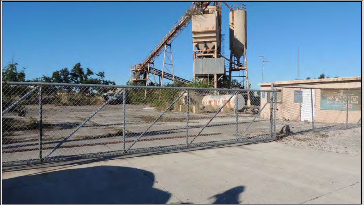
View from Seaboard Avenue Near Center
