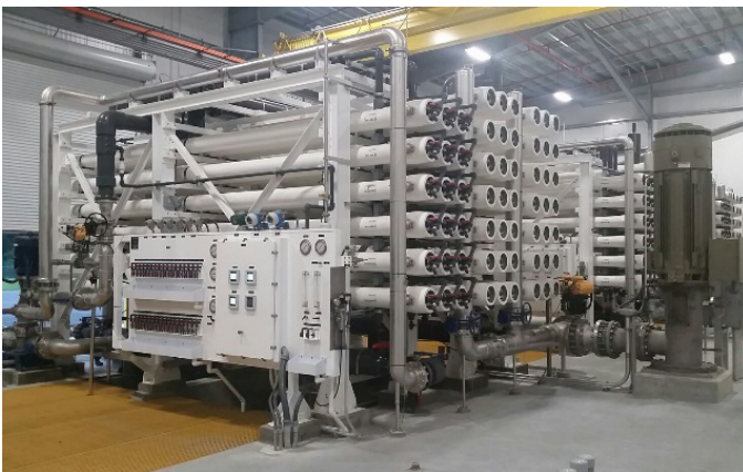
Jacobs provided services from RO Membrane Water Treatment technology to brackish groundwater wellfield development and concentrate disposal through UIC injection well.
