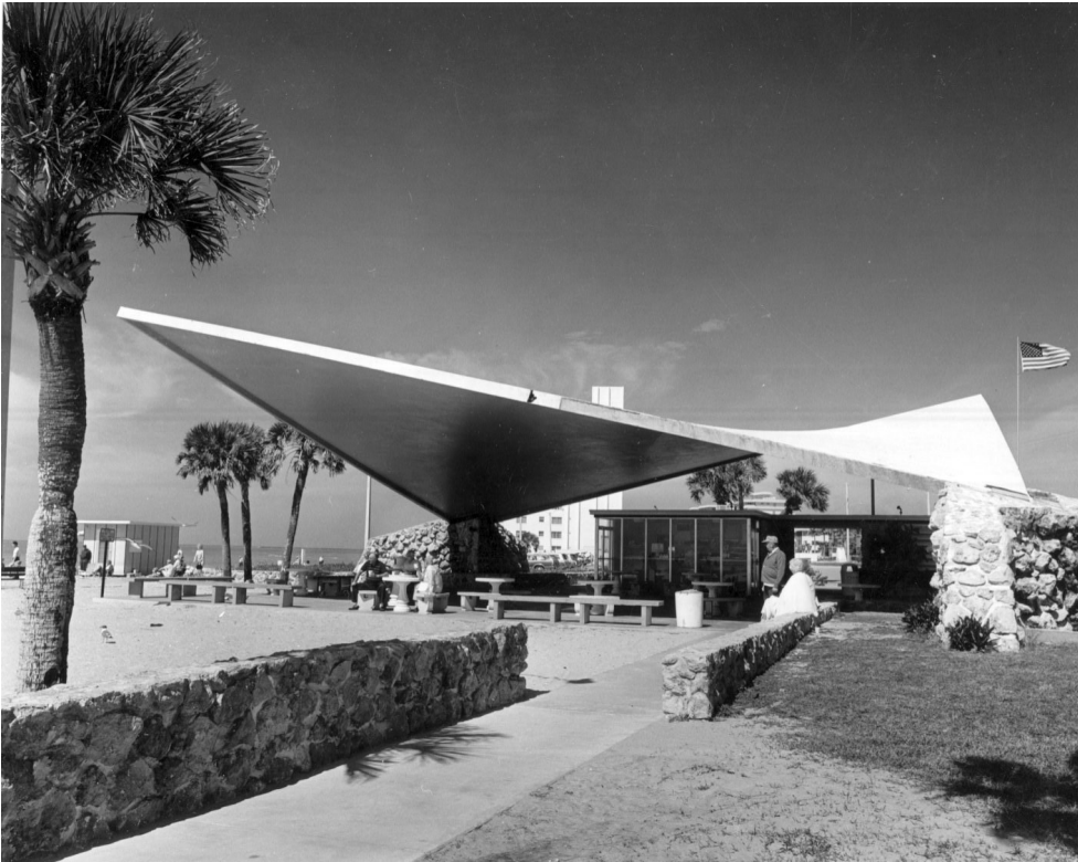
Completion of the Venice Beach Pavilion, January 1964.
