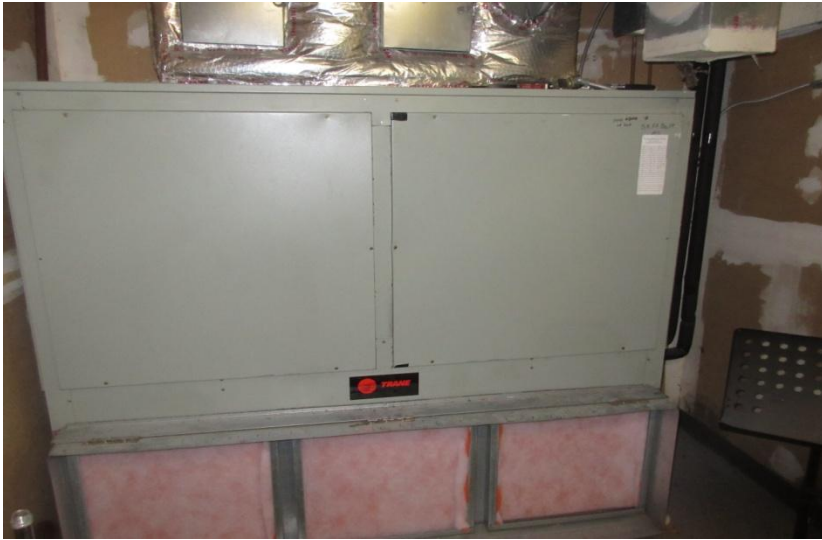
21) AHU-2 was assessed.
