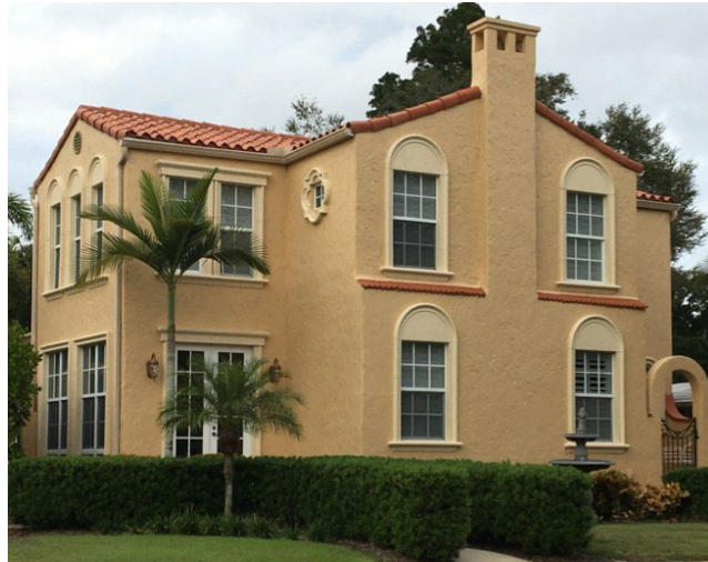
An exemplary two-story home built in 1926, 332 Ponce de Leon Ave. This is a simple design, with few elements: mullioned windows, all rectangular with about half having arches over them. It has a symmetric design, with the entry on the right
