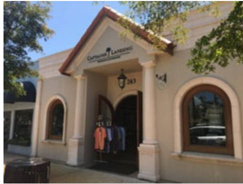
This building at 243 W. Venice Ave. is consistent with VHP principles: muted colors, trim slightly different from the fascia, simple arched windows, gracious entry. The single story is compatible with the narrow width so the vision is modest in scale.
