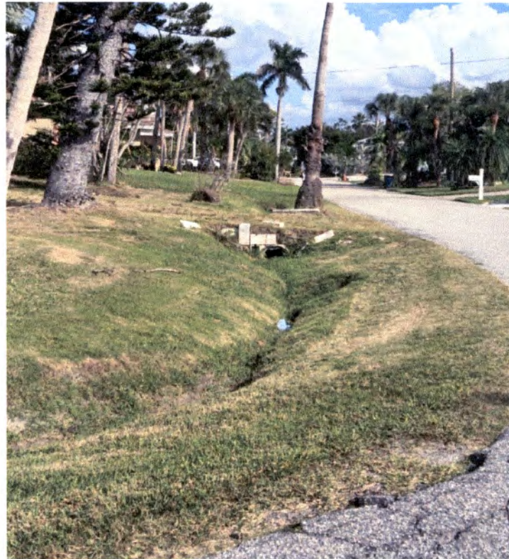
Figure 10: Swale at 397 Flamingo Drive in need of retrenching. Photo facing east.
