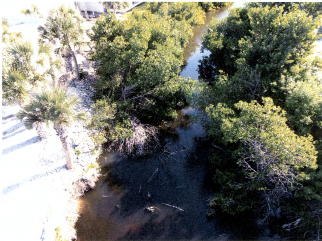
Figure 2: Vegetation blockages at "neck" of Flamingo Ditch. Photo facing east, just south of Island Shores (on left)
