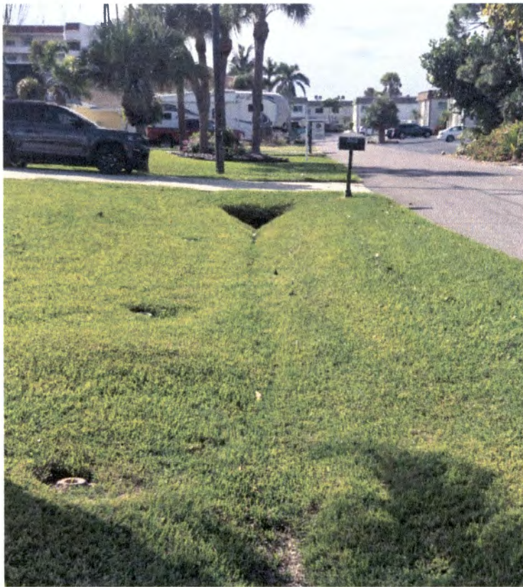
Figure 11: Swale needing retrenching at 593 Flamingo Drive. Photo facing west.
