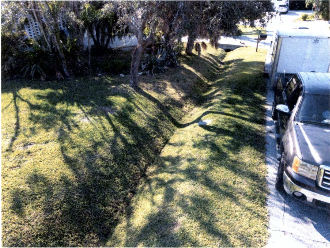
Figure 9: Retrenched swale in foreground, untrenched swale downstream at 397 Flamingo Drive. Facing south.
