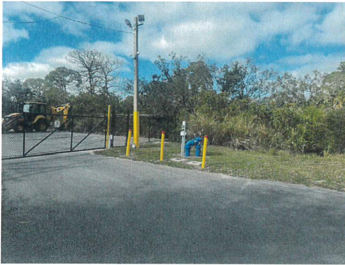
View looking at subject from parking lot
