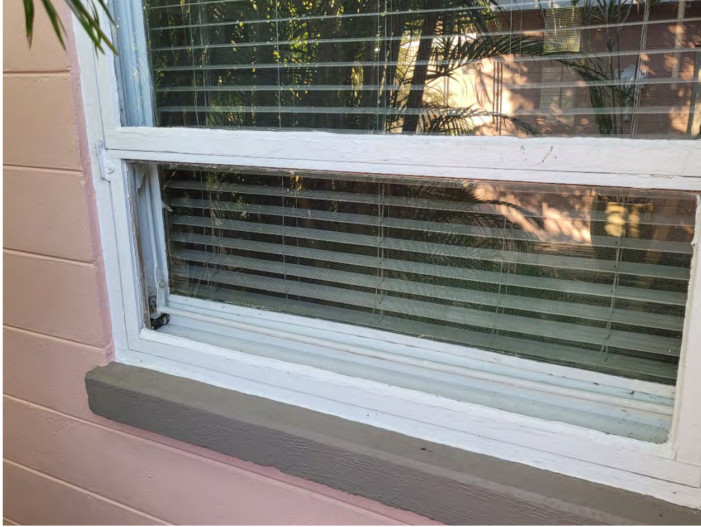
Figure 9 Detail of wood awning window showing mechanism.
