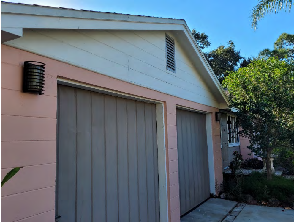
Figure 11 Two car garage built at the same time as the main house. Same architectural details, original garage doors. Faces Armada Rd.
