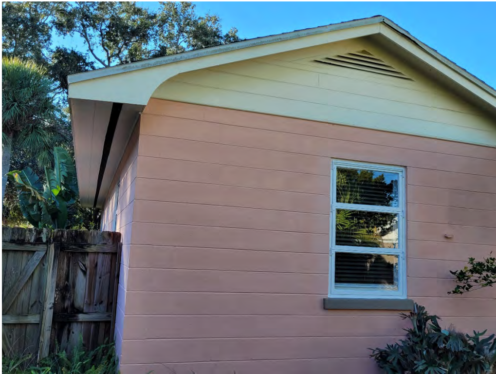
Figure 10 Rear gable end and wood awning window.
