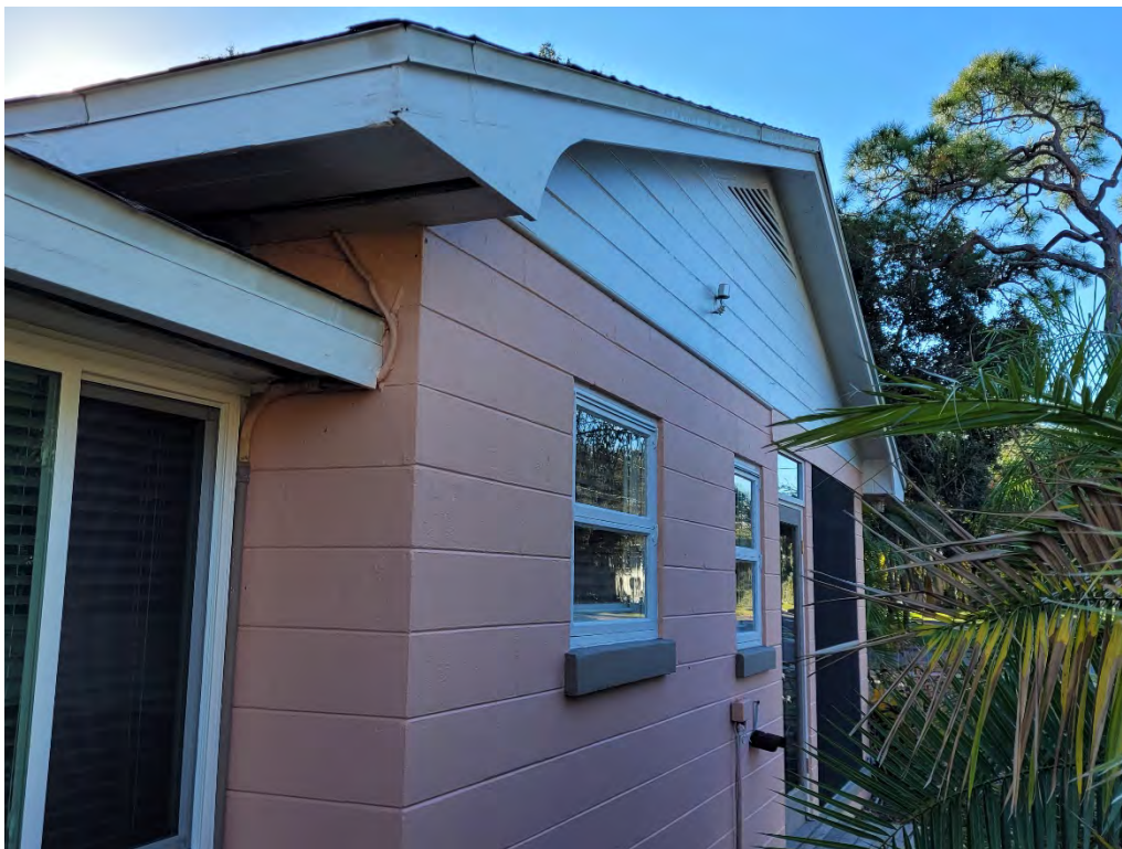
Figure 8 Armada Rd. gable end.
