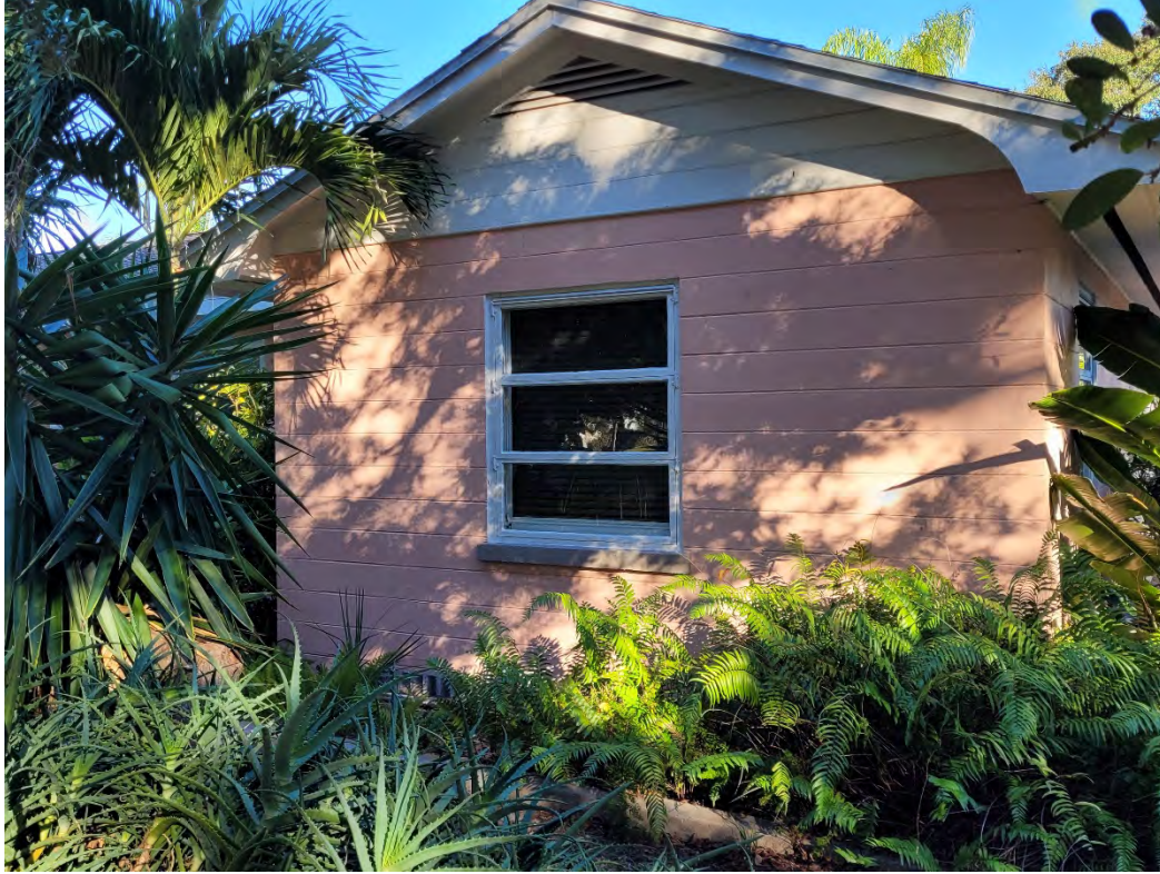
Figure 5 Detail showing wood awning windows; painted concrete block; wood gable end with wood attic vent; wood soffit with screen venting; fascia with rounded profile; and lower concrete block crawlspace
