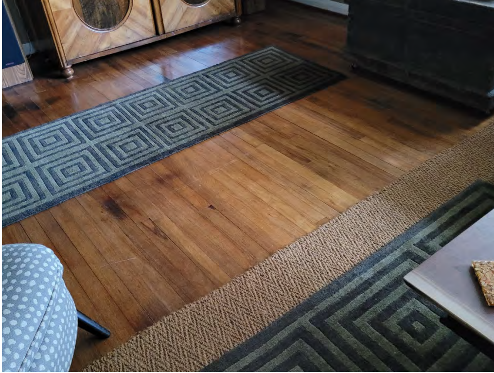
Figure 23 Detail of unrestored oak flooring in living room.
