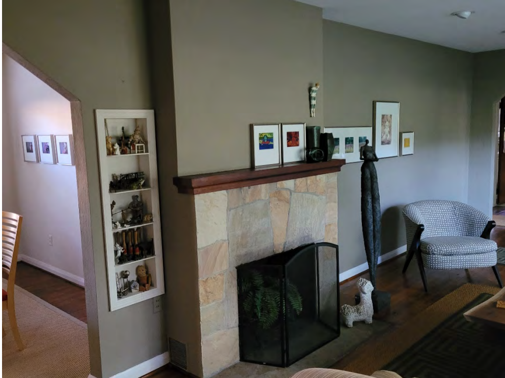
Figure 17 Living room detail showing original fireplace, hearth and mantle; original baseboards and unrestored oak floors.
