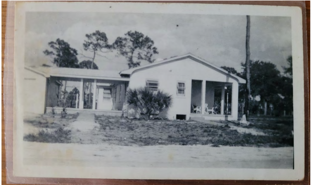
Figure 3 1948 image of house taken from Armada Rd. Shows open breezeway and porch, as well as crawlspace vent and access
