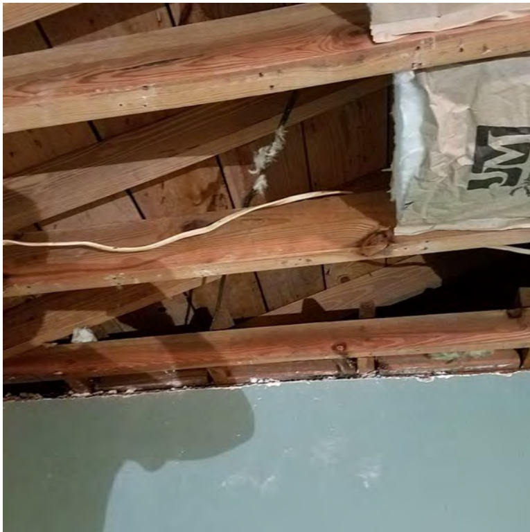
Figure 12 Roof construction detail showing 16" centers; 1" lumber decking; and what appears to be yellow pine true dimension trusses. Exposed during ceiling repair in bedroom
