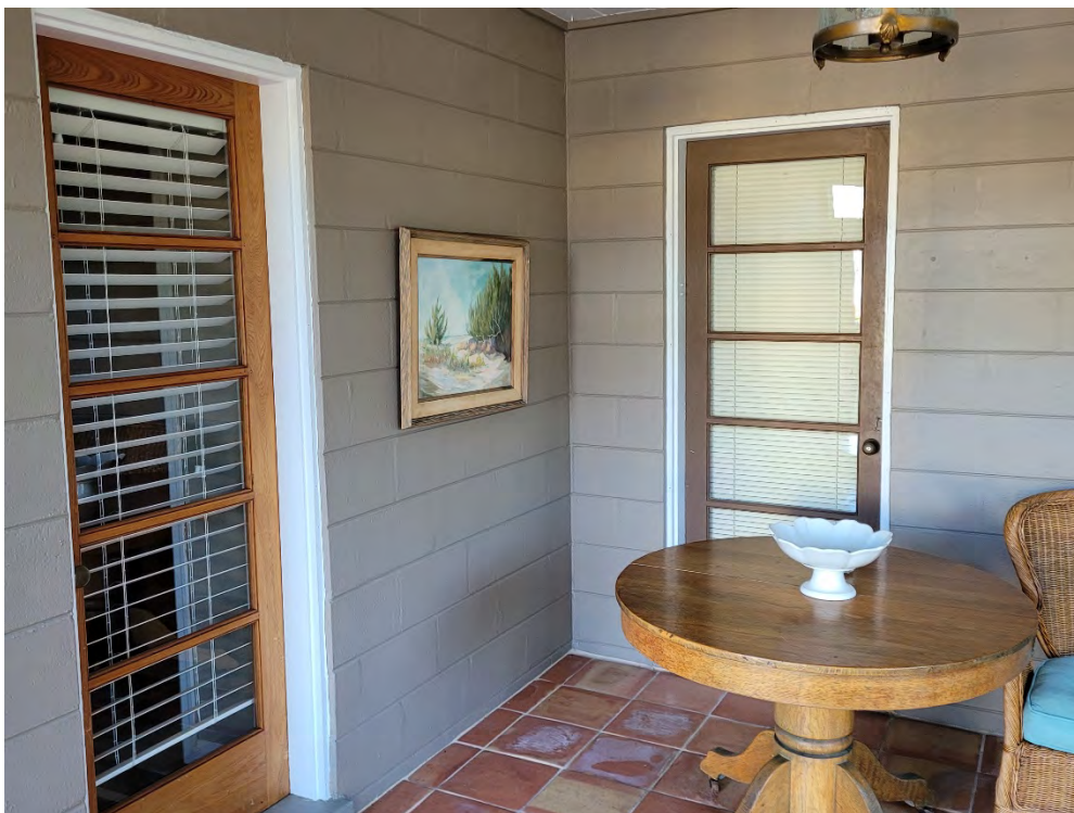
Figure 20 Interior of porch showing painted concrete block and original 5-light doors.
