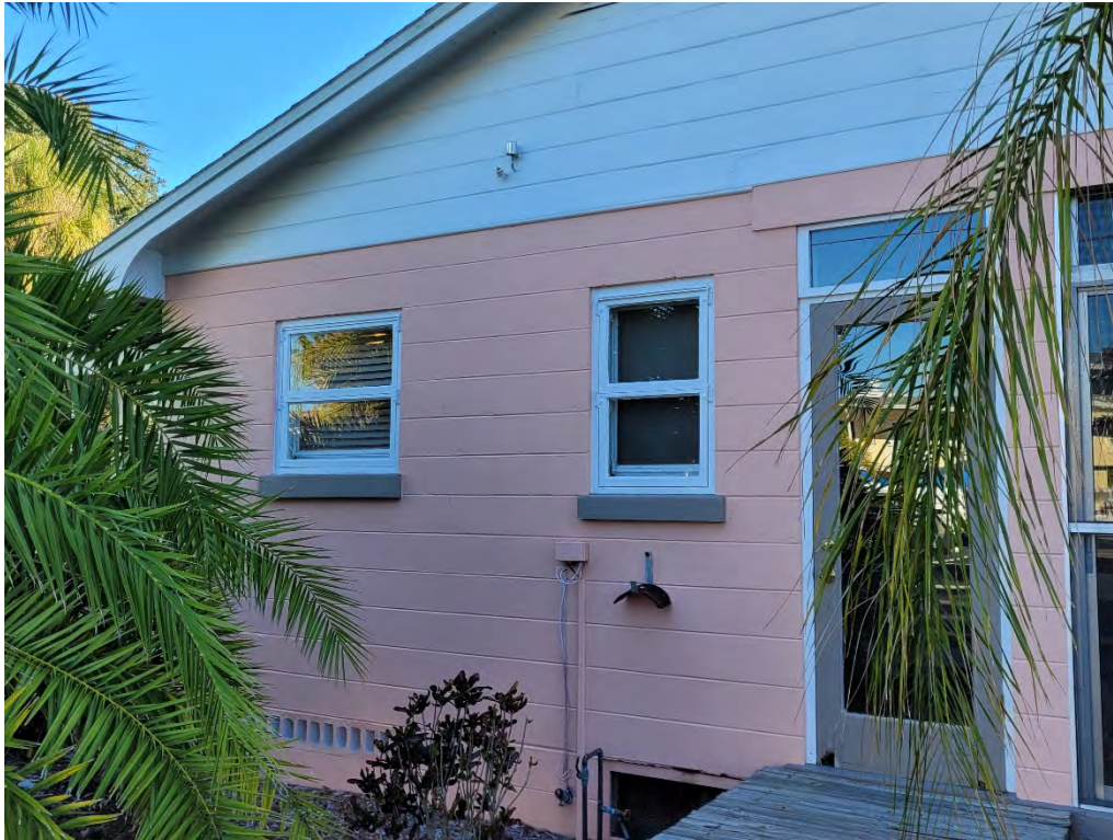
Figure 7 Detail with crawlspace vent and access panel, as well as previously listed structural elements.
