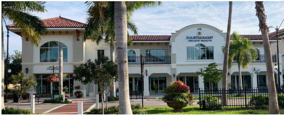
This photo is also of a new building at 310 W. Venice Ave. The massing of the structure is broken up by presenting two distinct façades, the larger, rightmost being symmetric and itself broken into three parts. The six first-floor openings are exact VHP.
