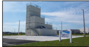
Fire Training Academy - Training Tower Completed 2015 ($660,000) Charlotte County
