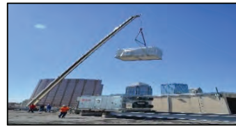
700 Twiggs Street Administrative Offices HVAC Improvements Completed 2017 ($1,200,000) Hillsborough County
