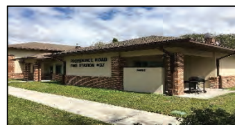
Fire Rescue No. 37 Providence - HVAC Renovation In Construction Phase 2018 (127,940) Hillsborough County
