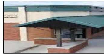
Wauchula Police Headquarters and New City Hall Completed 2003 (6,200 sq. ft.; $1,000,000) City of Wauchula
