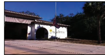
West Hillsborough Fire Station No. 31 - HVAC Replacement Completed 2013 (3,000 sq. ft.; $150,000) Hillsborough County
