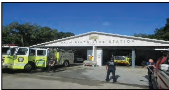
Fire Station No. 15 Palm River - HVAC Improvements Completed 2016 (3,340 sq. ft.; $127,380.00) Hillsborough County
