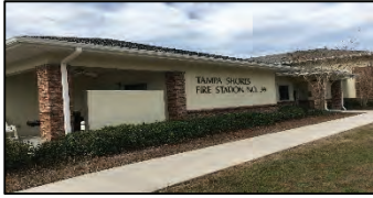
Fire Rescue No. 39 Tampa Shores - HVAC Renovation Completed 2018 (46,980) Hillsborough County
