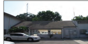
Brandon Fire Station No. 11 - HVAC Replacement Completed 2013 (7,500. sq. ft.; $258,909) Hillsborough County
