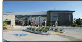
Pasco Data Center and Supervisor of Elections New Service Center Completed 2014 ($10,145,000) Pasco County Board of County Commissioners
