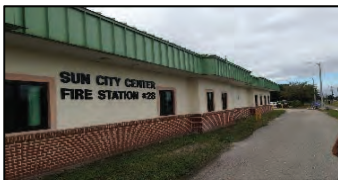
Fire Station No. 28 Sun City Center - HVAC Improvements Completed 2016 (4,500 sq. ft.; $127,380) Hillsborough County
