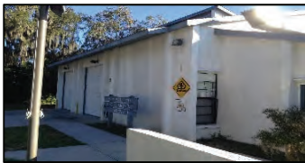
Fire Station No. 30 Midway Plant City HVAC Improvements Completed 2016 (2,760 sq. ft.; $64,680.00) Hillsborough County
