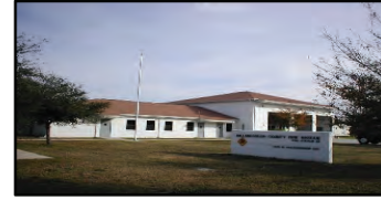
West Hillsborough Fire Station No. 20 - HVAC Replacement Completed 2013 (6,500 sq. ft.; $99,000) Hillsborough County
