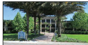
Municipal Complex Emergency Power Improvements In Construction 2018 ($2,000,000) City of Largo
