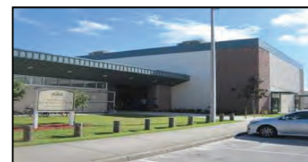
Northwest Multi-Purpose Gymnasium @ Westchase Community Center Completed 2014 (9,000 sq. ft.; $1,674,000) Hillsborough County
