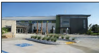
Pasco Data Center and Supervisor of Elections New Service Center Completed 2014 ($10,145,000) Pasco County Board of County Commissioners
