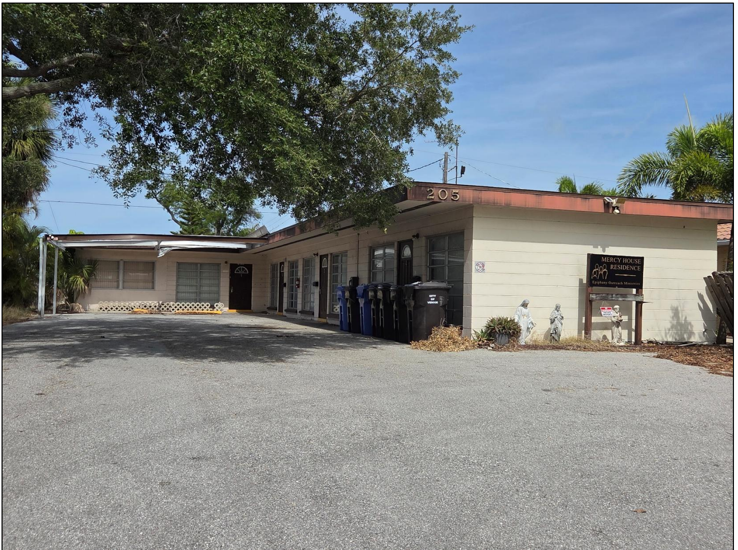
Existing 1959 building to be demolished
