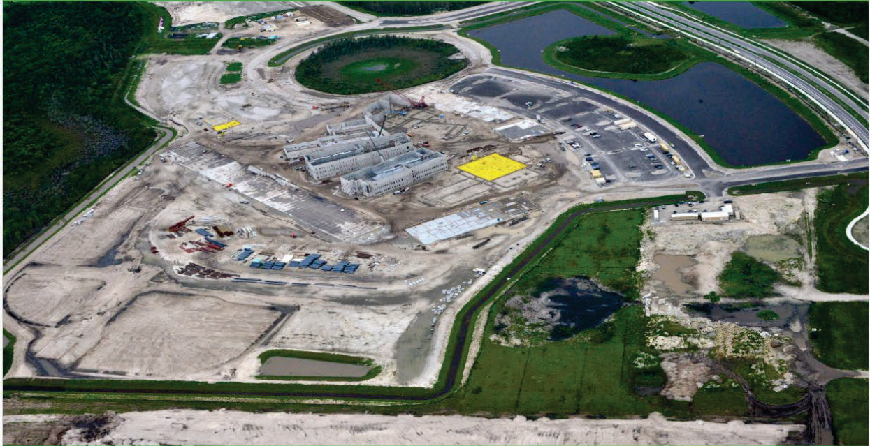
Wellen Park HS—Under Construction
