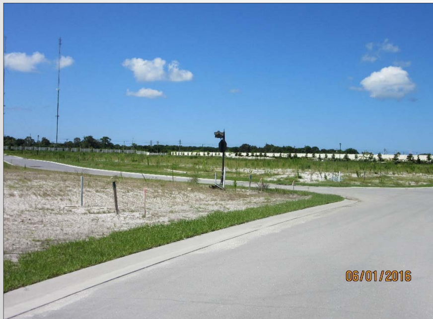
View of Unit 1, Phase 4 looking south toward Laurel Road. Pescador Place is the street in the foreground.
