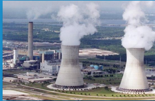
St. Johns River Power Park (FPL/JEA joint ownership) Officially retired in early January 2018
