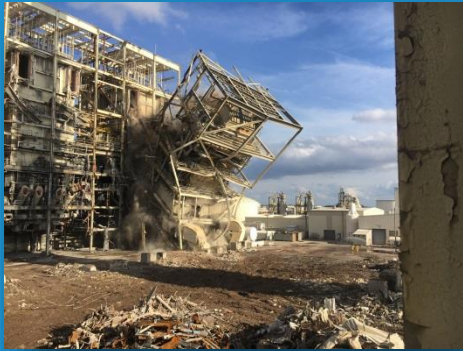
Cedar Bay coal plant Demolition underway
