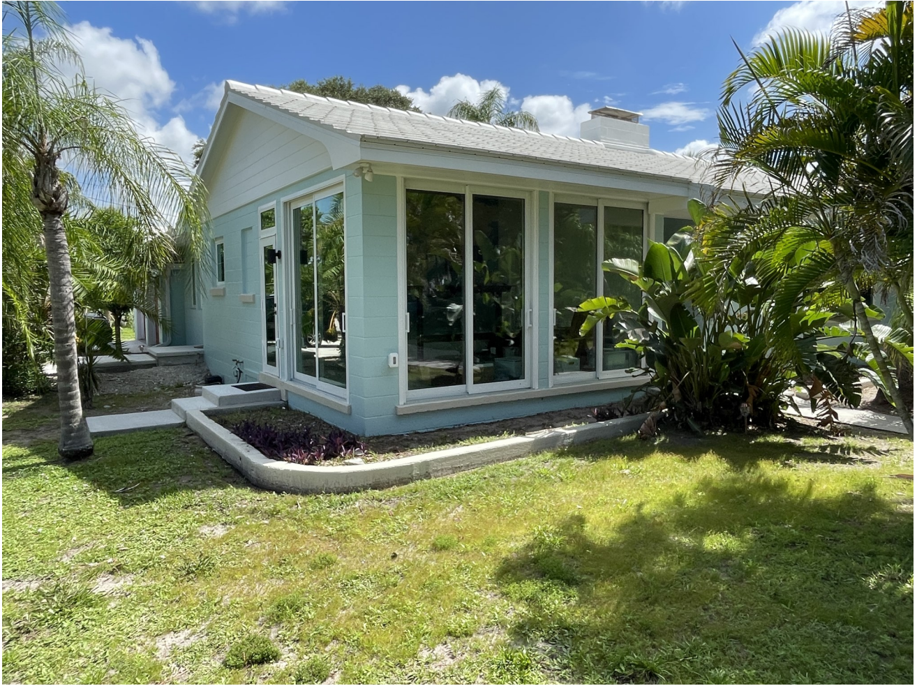
Enclosed front porch.
