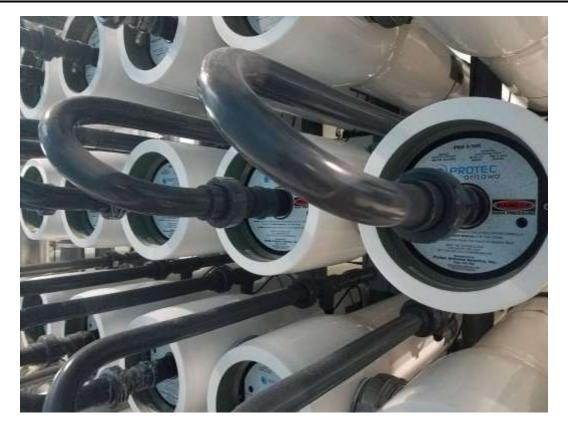
Figure 3: RO Permeate Collection from Pressure Vessels
