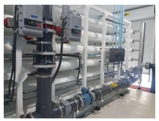
Figure 2: RO Membrane Skids and Concentrate Pipe Line
