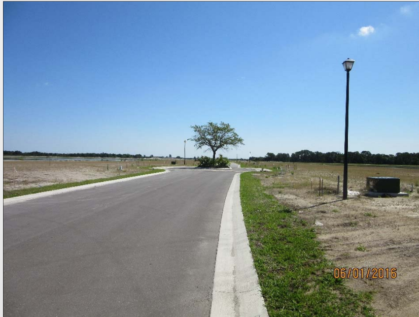
View looking northeast along Toscavilla Blvd. toward area of proposed Unit 2
