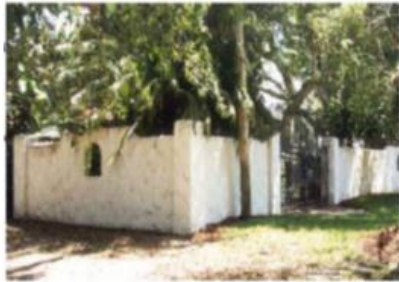
Figure 7.10.9. Fences and Walls
