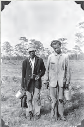
Turpentine industry workers, ca. 1930s
