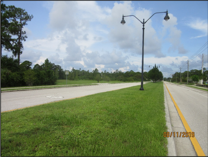
West along Border Road, Sarasota County stormwater pond is on the left
