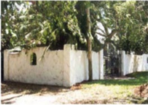
Figure 7.10.9. Fences and Walls
