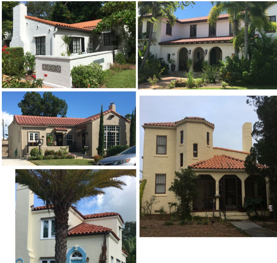
Examples of Permitted Roof Materials in Use
