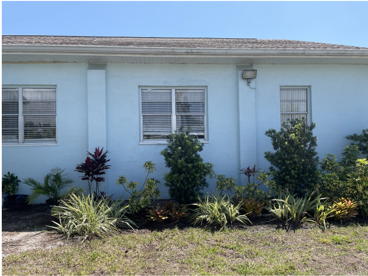
West end of front façade looking south.
