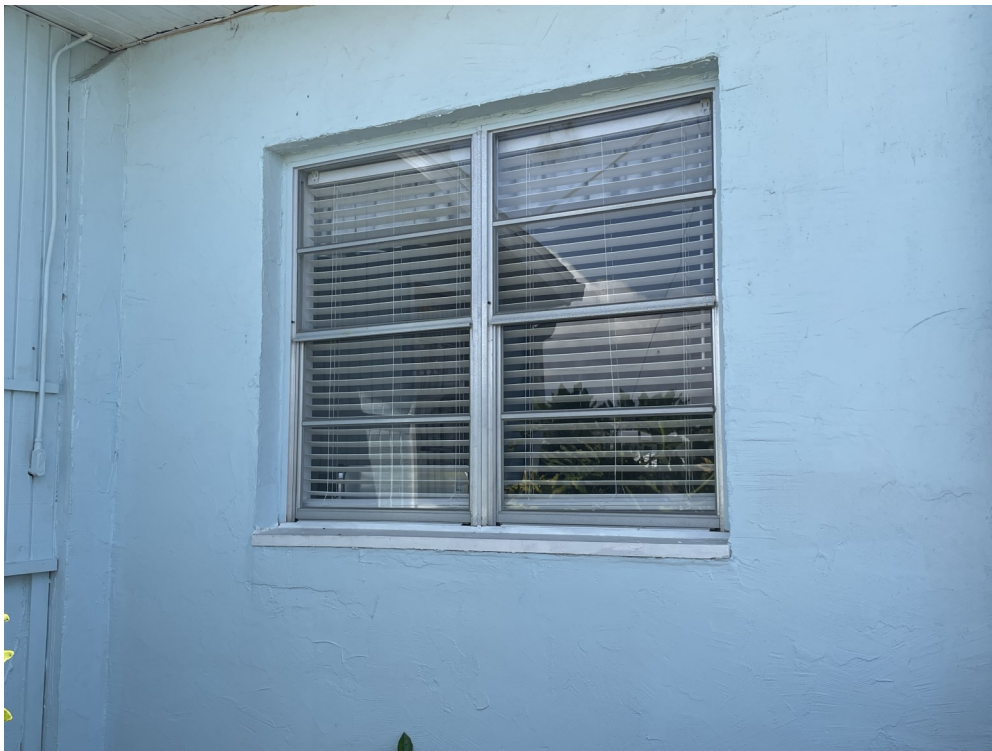
Close up of replacement window on front façade.
