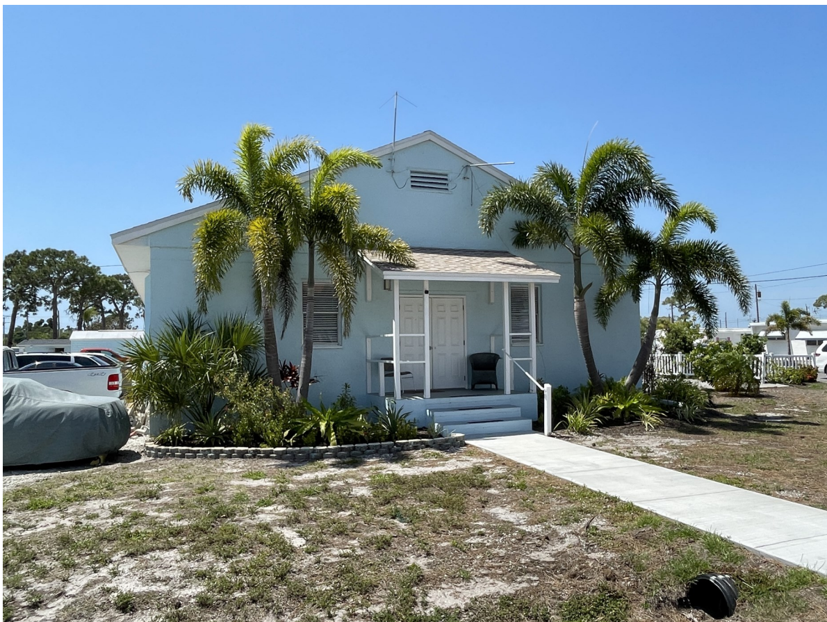
East façade looking west
