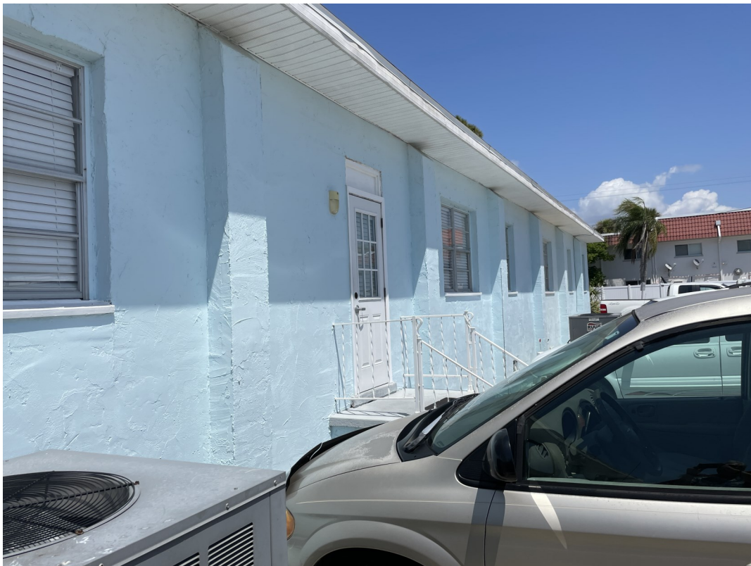
Rear of building looking northeast.
