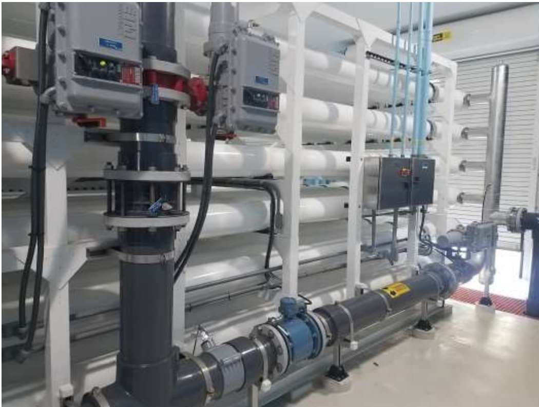
Figure 2: RO Membrane Skids and Concentrate Pipe Line
