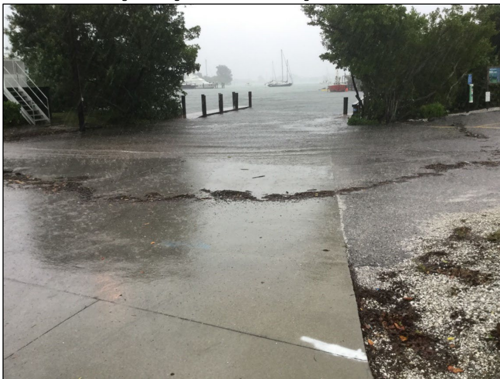
Figure 1: Higel Marine Park Flooding
