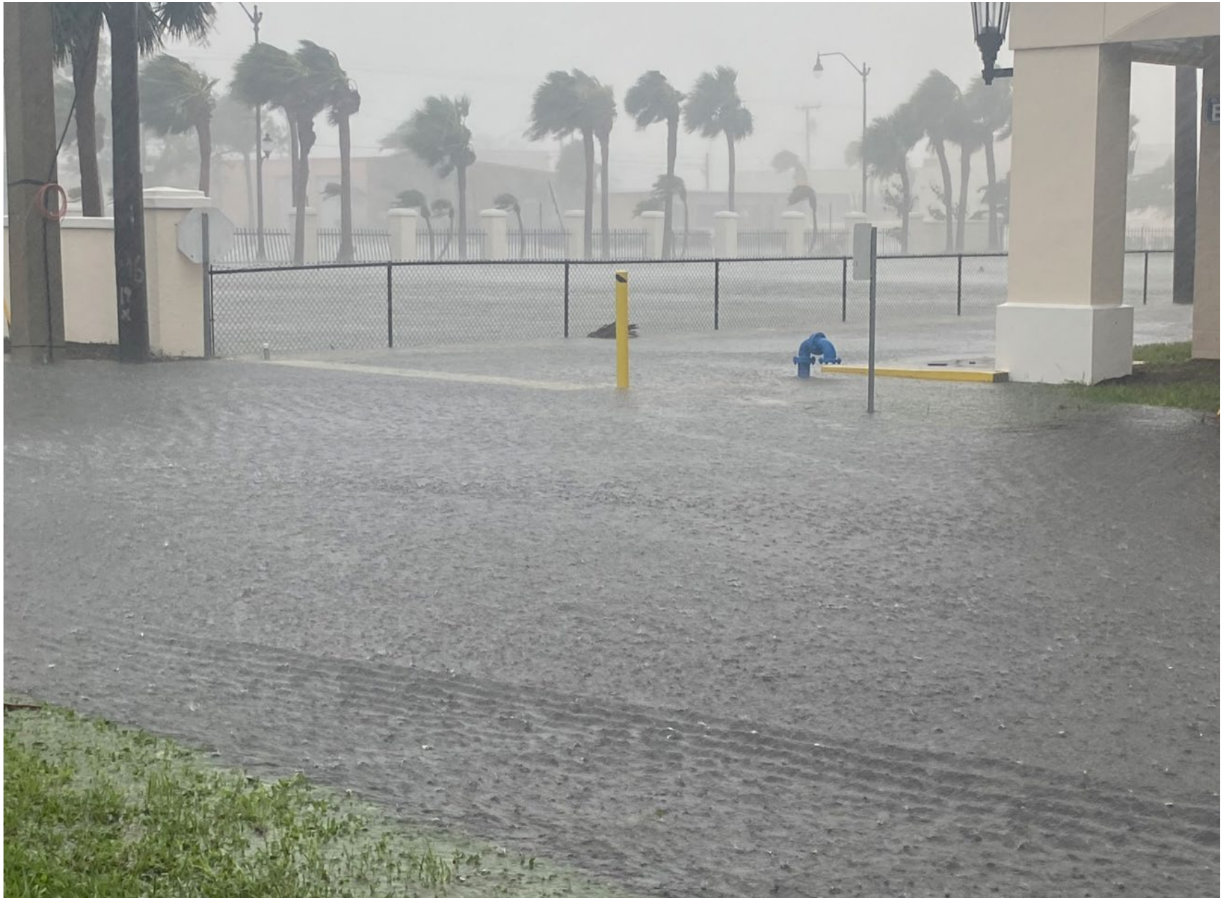
Water Treatment Plant Area during Hurricane Ian (Sept. 2022)
