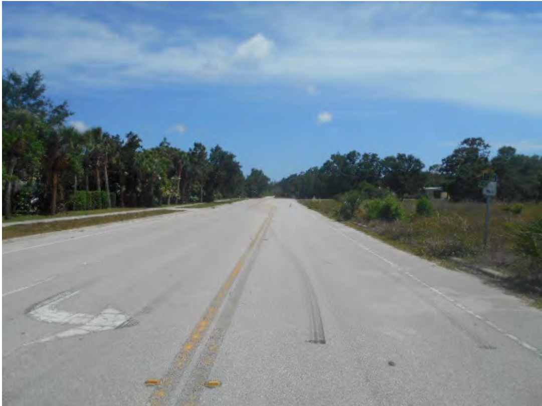
Street acene looking south along Auburn Road from Venice Avenue with subject to right
