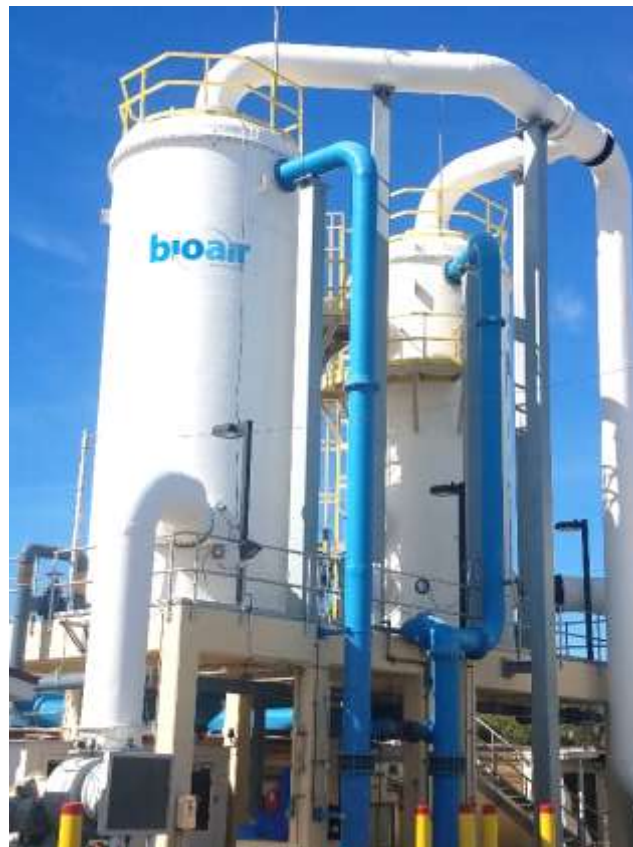
Figure 4: Forced Draft Degasifiers to Remove Hydrogen Sulfide from Finished Water
