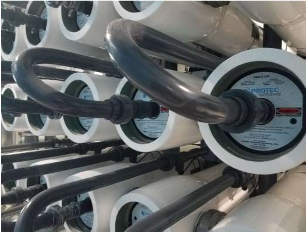
Figure 3: RO Permeate Collection from Pressure Vessels
