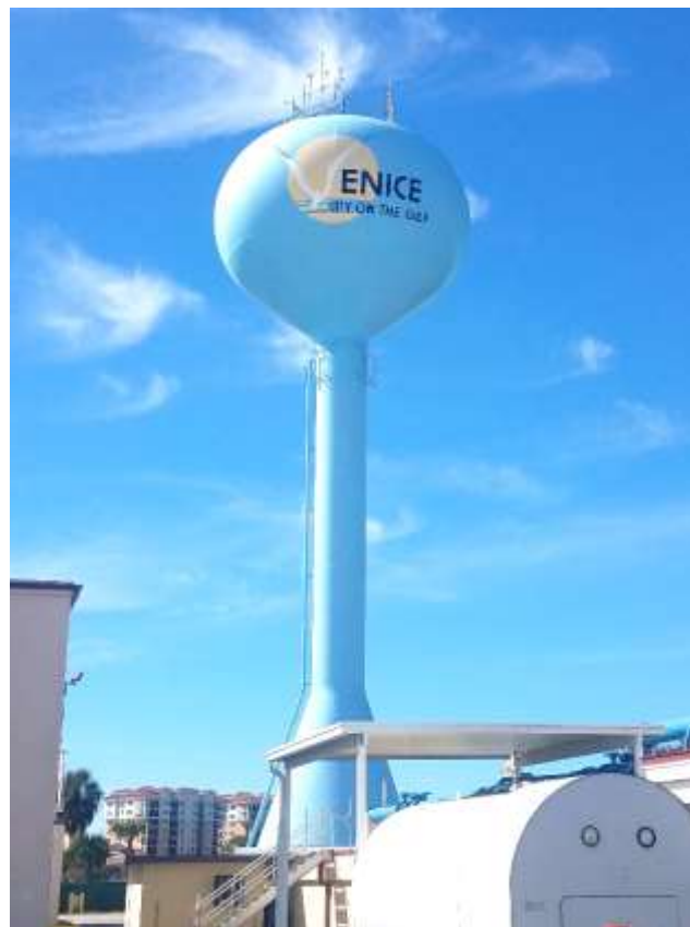
Figure 5: Elevated Water Storage Tank at WTP Site
