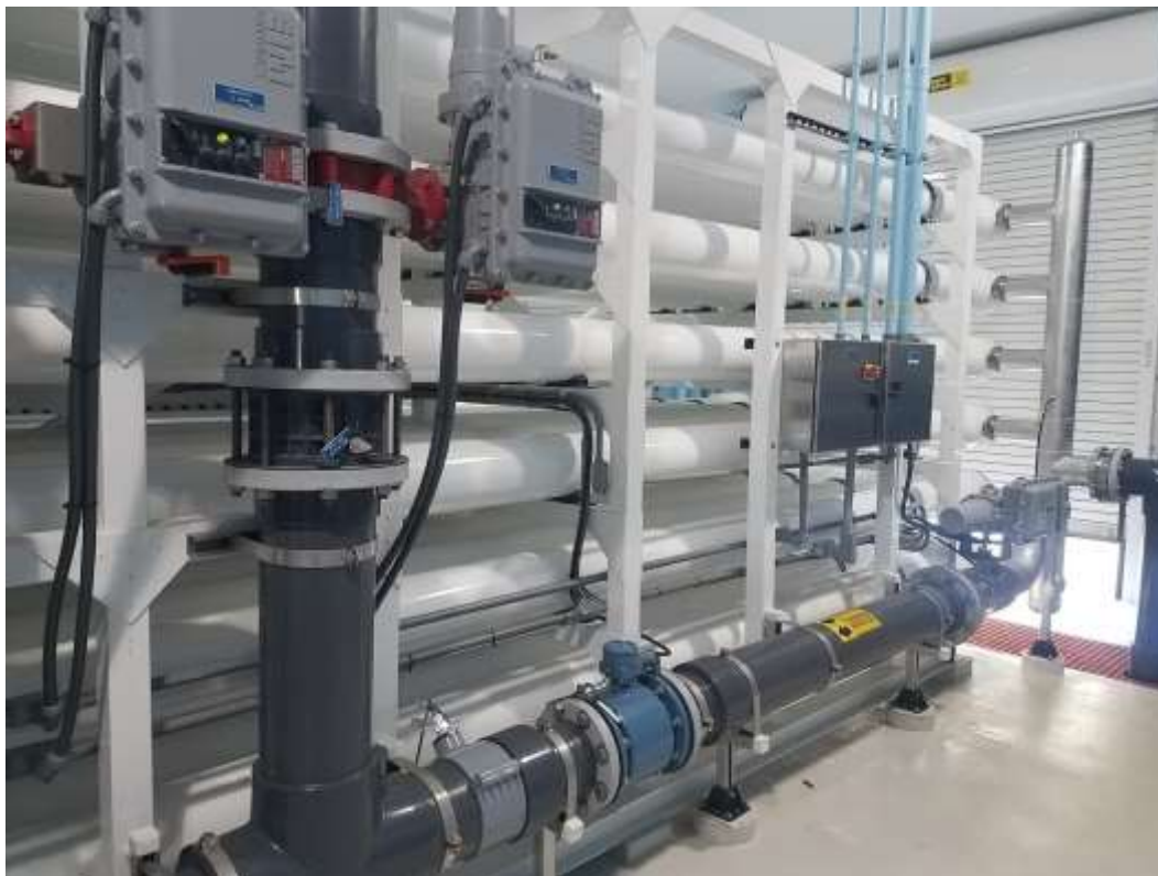
Figure 2: RO Membrane Skids and Concentrate Pipe Line
