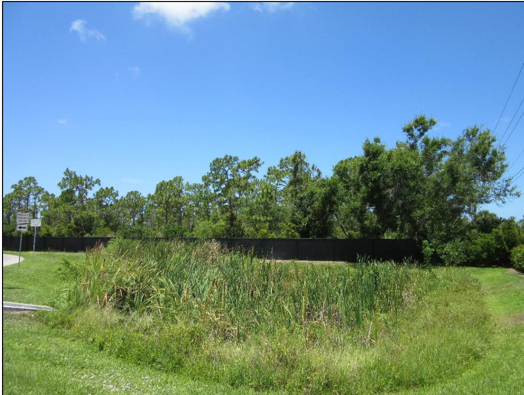
View from Venice Police Department along eastern property line
