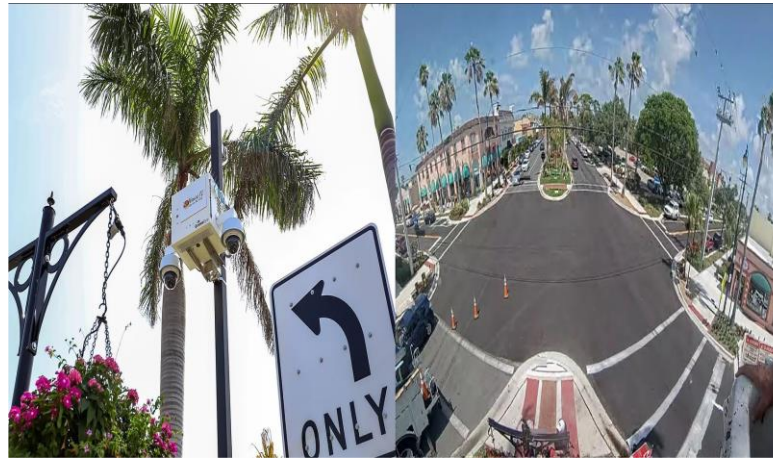
Security Camera System
