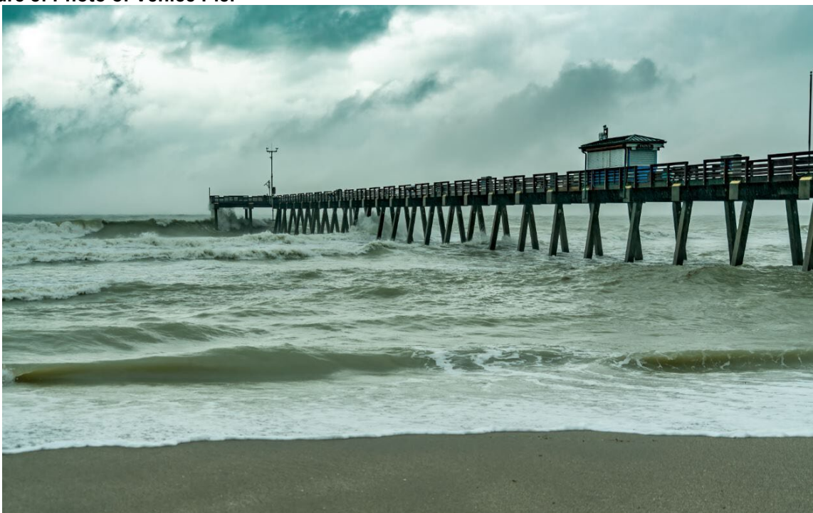
Figure 8: Photo of Venice Pier
