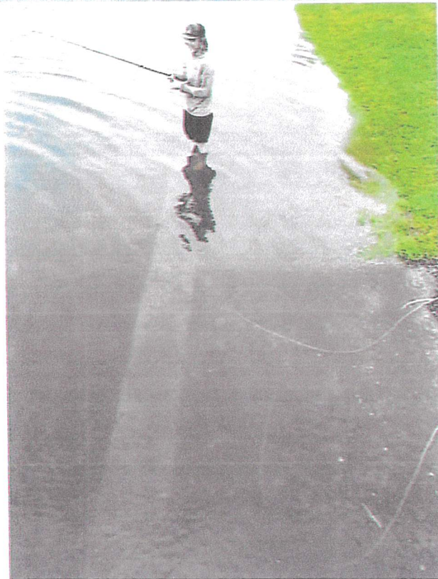
Images illustrating Seawall Width & Overflow Height of 2 ft plus for most of August 2024
