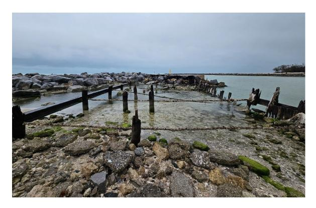
The hurricane impact severely damaged both the rock revetment and bulkhead infrastructure and caused major erosion of portions of the site interior. With this critical navigational structure compromised, any delays in enacting a plan of restoration creates a greater threat to the Venice Inlet channel itself. An FY26 appropriations request has been submitted for \$100 million in USACE funding.
