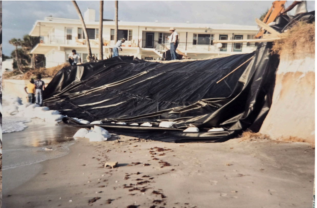
Beachcomber seawall reinforcement measures
