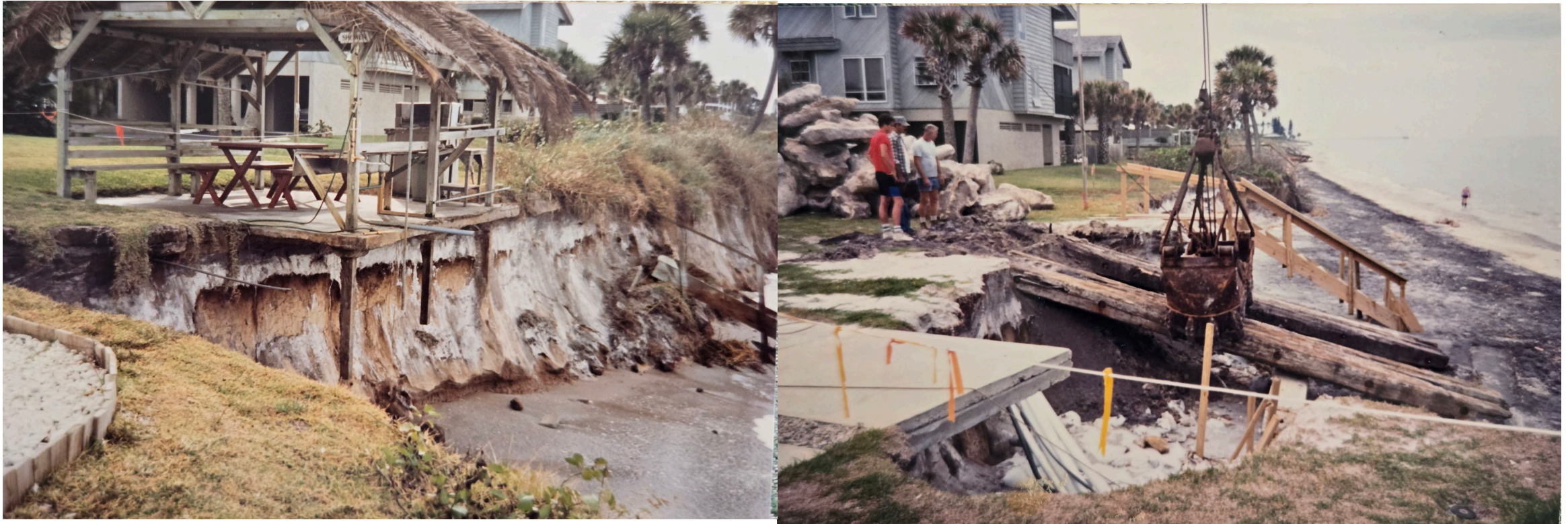
Beachcomber erosion control Measures – before the Renourishment Program
