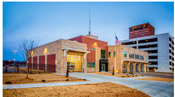
Bartlesville Police and Municipal Fire Complex
