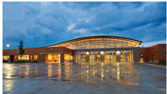
Travilah Fire Station No. 32
