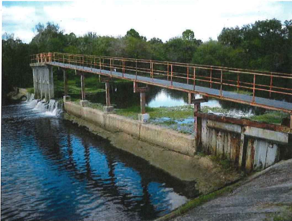
Old Water Control Structure No. 101
