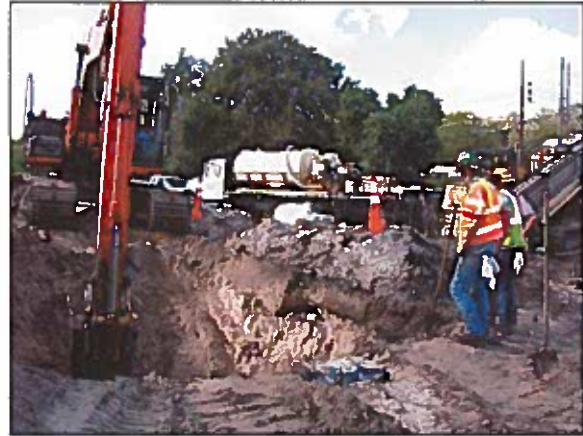
Bore Hawg Pit Excavation for 20" Install
