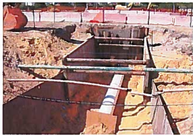
Killebrew Construction's 30" Slipline
