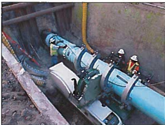
Garney Construction's 30" Slipline
