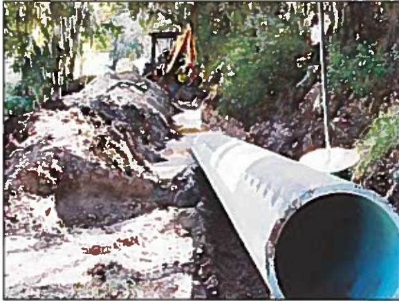
Bore Hawg's 20" Install
