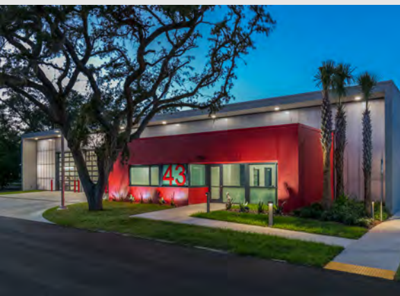
LARGO FIRE STATION #43 BELLEAIR BLUFFS, FL
