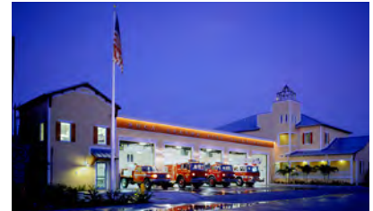
Boca Grande Fire Department, Boca Grande, FL
