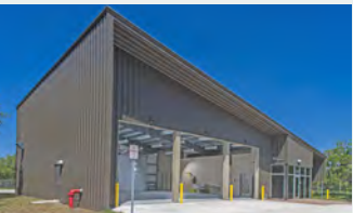
2014 Brighton Forestry Fire Station Brighton, FL
