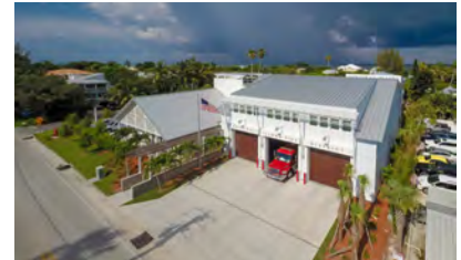
Captiva Island Fire Station Captiva, FL
