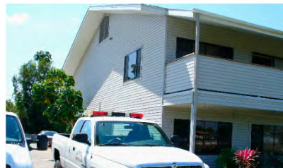
Pine Island Fire Station #1 Remodel Pine Island, FL
