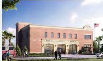
2018 Immokalee Fire Station #31 Immokalee, FL
