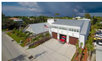
2015 Captiva Island Fire Station Captiva, FL
