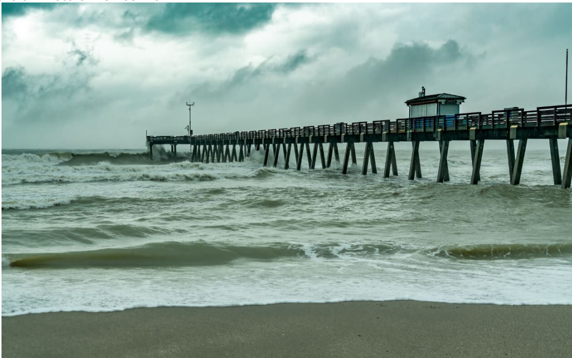
Figure 8: Photo of Venice Pier
